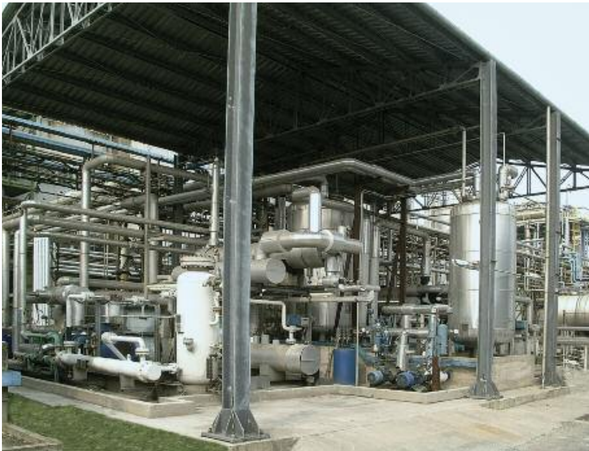
-70°C refrigeration system for antibiotics production.
