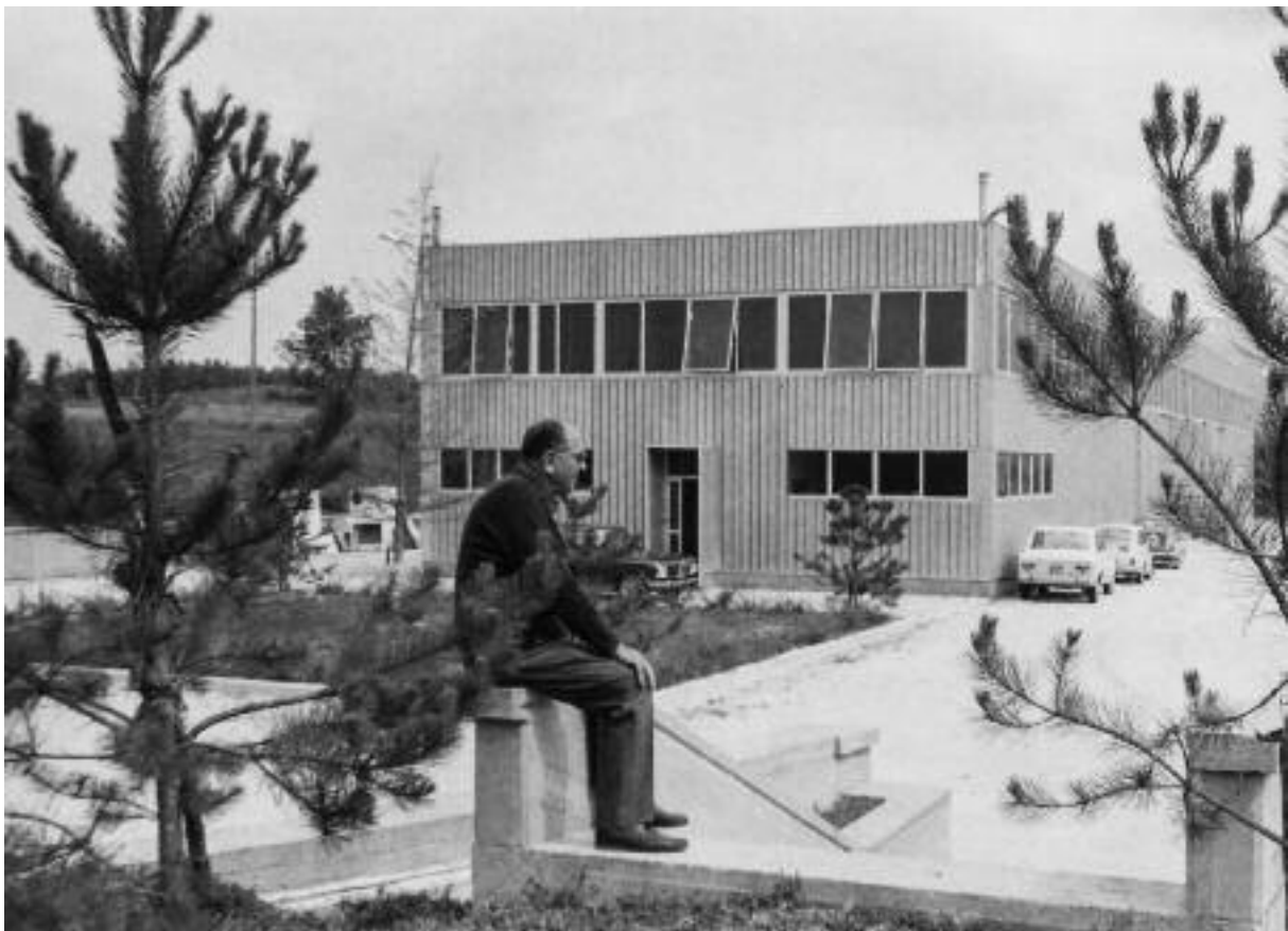
The construction begins of the ACS plant in Cimacolle, Massa Martana, 1968.
