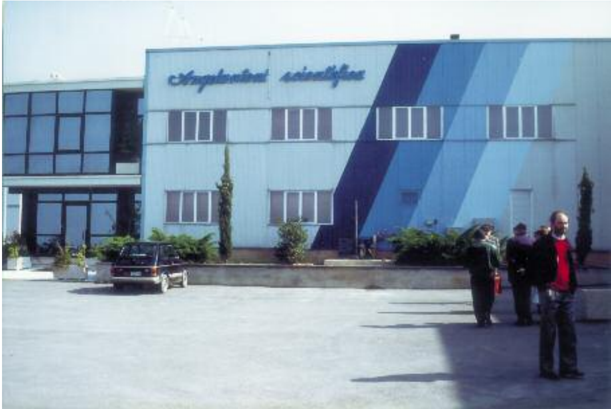
Angelantoni Scientifica office block and plant in Massa Martana.
