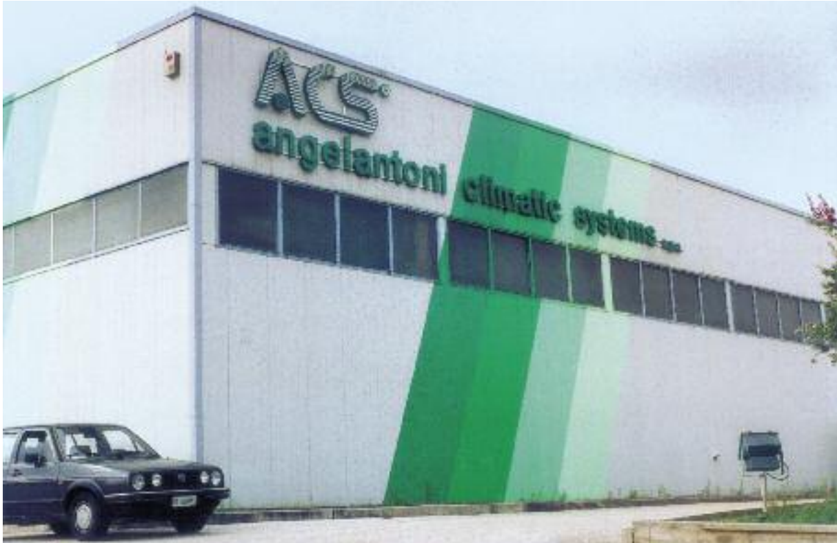
The new ACS plant in Massa Martana.
